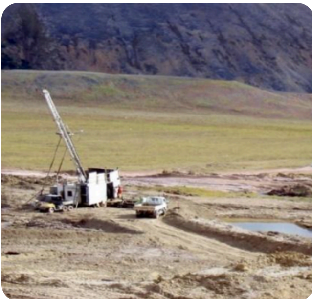
Fig. 2. Drilling of inclined wells
